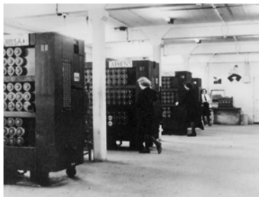
Bombe Control Room
